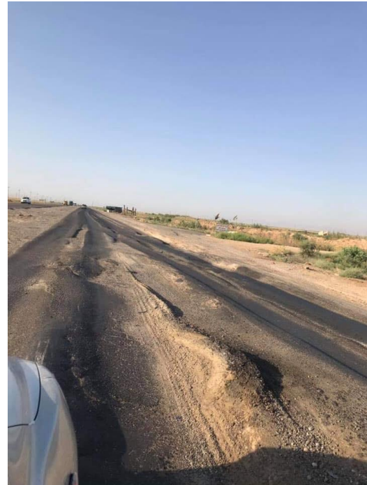
Figure 5. A photograph depicting a damaged section of the highway with visible cracks and potholes caused by heavy tanker truck movement.
